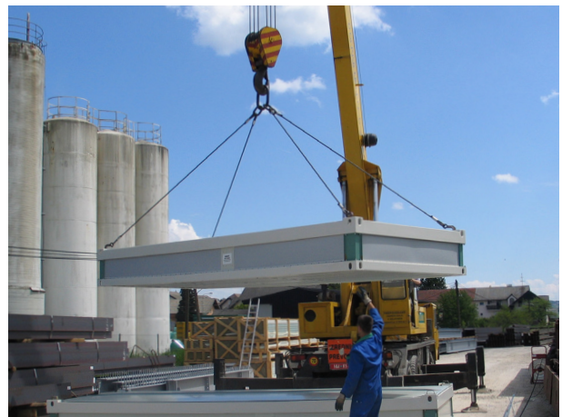
Handling of modular units with crane
